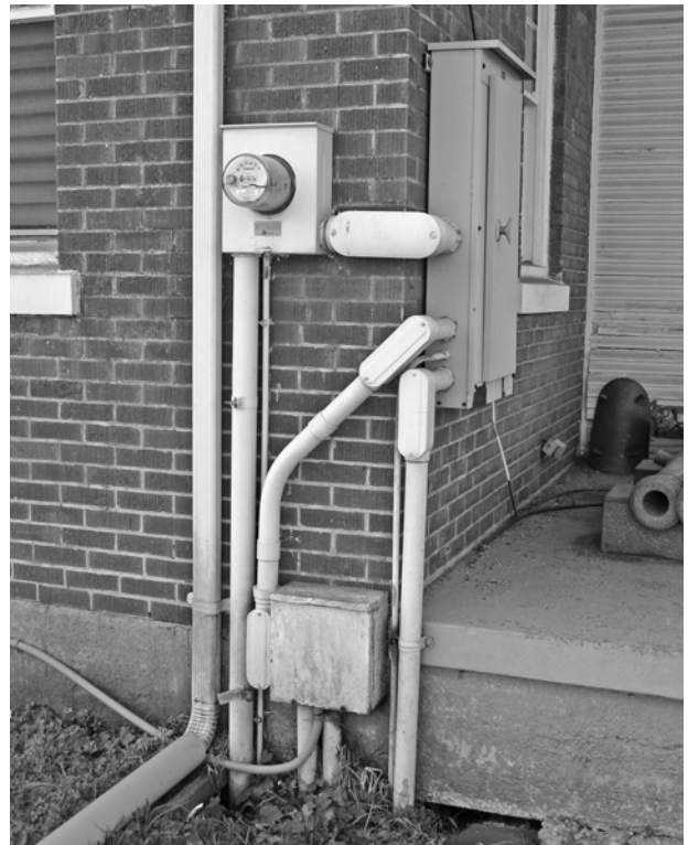
FIGURE 63. View of electrical service at north corner of house.
