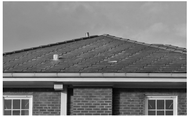
FIGURE 47. View of southwest shed of main roof.
