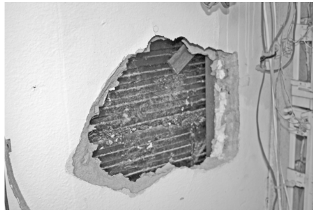
FIGURE 32. View of water-proofed interior face of structural clay tile walls behind plaster-board walls.
