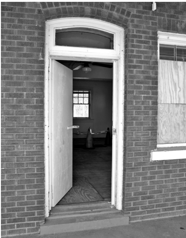
FIGURE 41. View of one front door.
