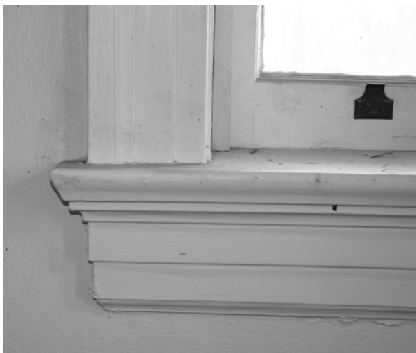
FIGURE 62. View of typical window casing and stool.
