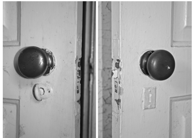
FIGURE 59. View of typical original interior door hardware.
