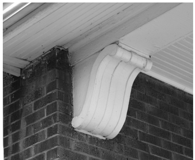
FIGURE 44. View of front porch eave and console.
