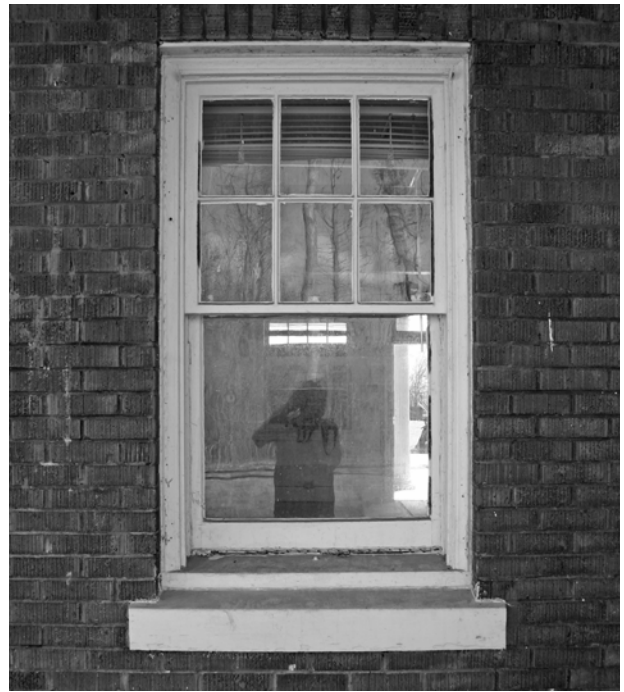
FIGURE 37. A typical 6/1 window.
