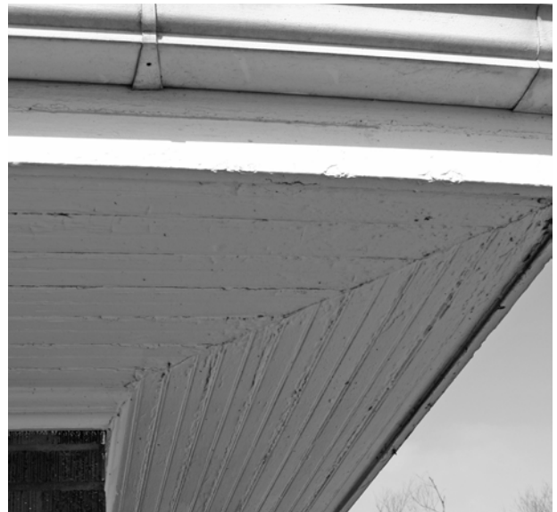
FIGURE 43. View of southeast corner of eaves on main block.
