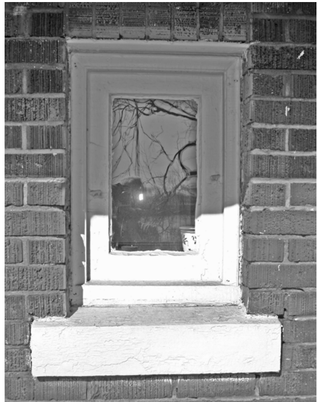
FIGURE 31. View of wood-framed window with typical cast-iron angle-iron lintel and cast-stone sill.
