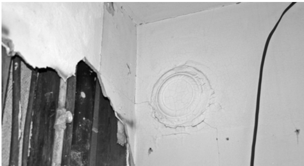
FIGURE 67. View of original stove flue in south corner of Room 103.
