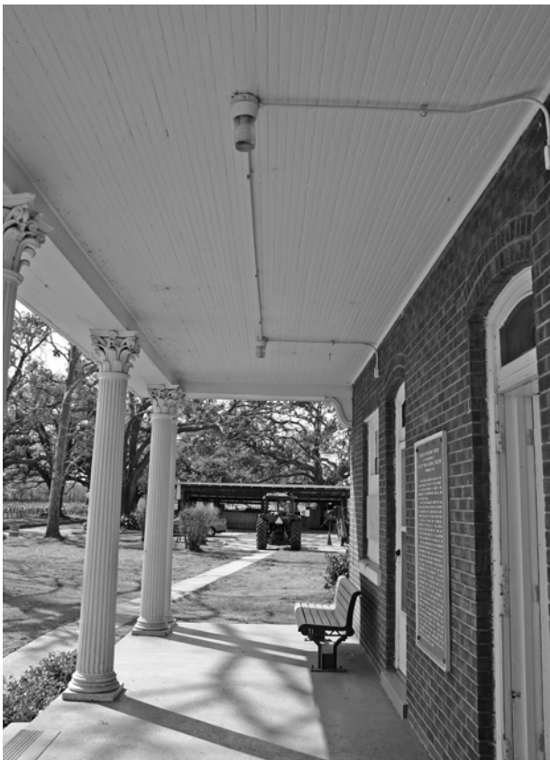
FIGURE 36. View southwest on front porch.
