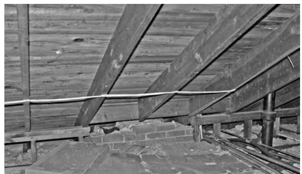
FIGURE 33. View of attic framing.
