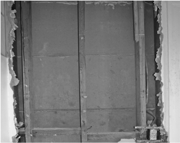
FIGURE 56. View of wall in Room 103 with rock lath in adjacent room exposed.
