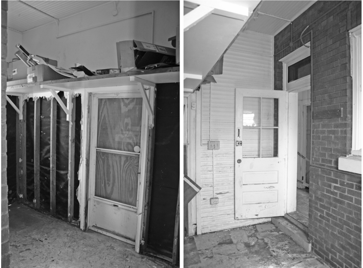
FIGURE 72. View west (left) and east (right) in Room 106.
