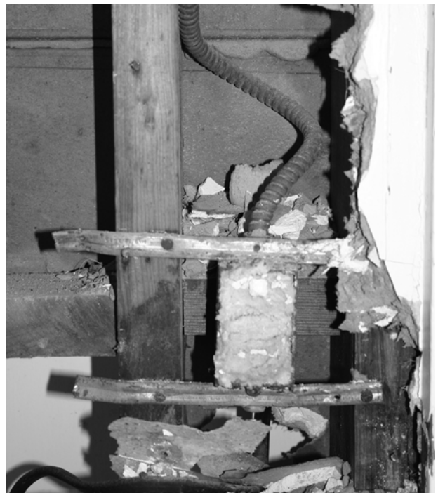
FIGURE 64. View of original switch box and BX electrical cable, abandoned in 1965.
