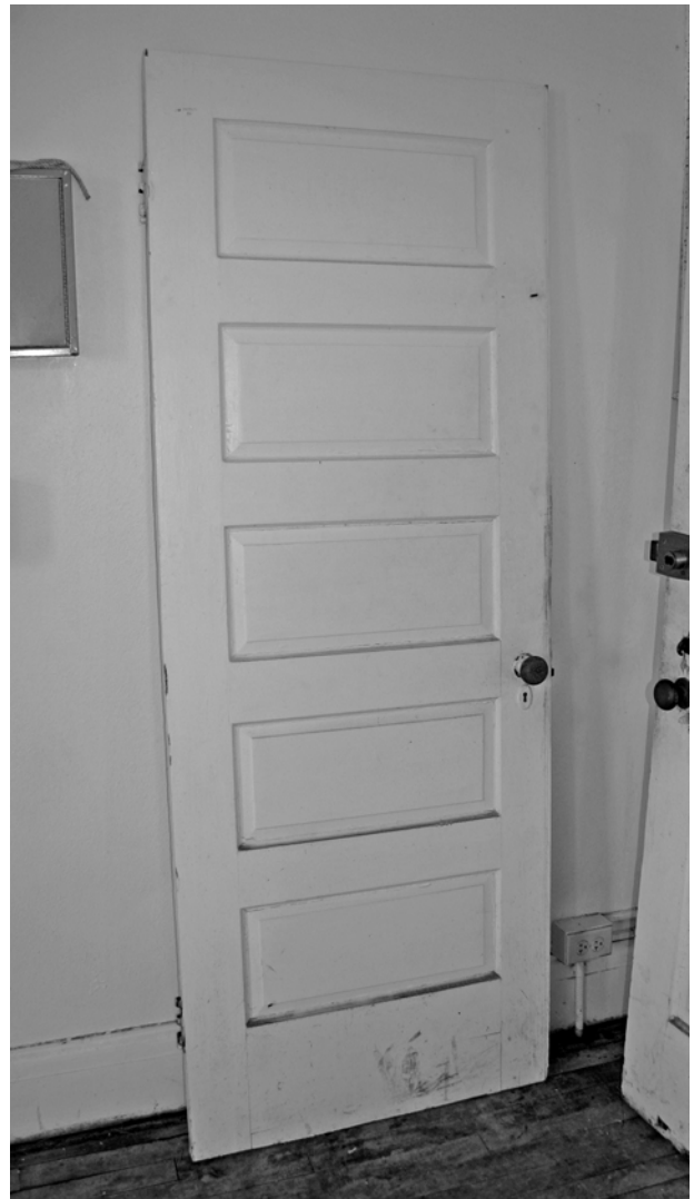
FIGURE 58. View of typical original five-panel interior door.
