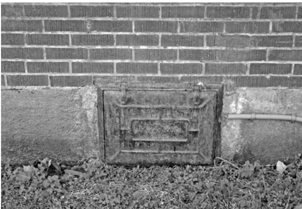
FIGURE 30. View of altered foundation opening on northeast side of house.
