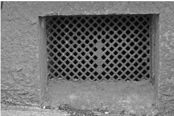
FIGURE 29. View of typical porch foundation vent.
