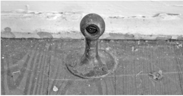
FIGURE 60. View of typical door stop, minus some sort of rubber feature that would have filled the hole.
