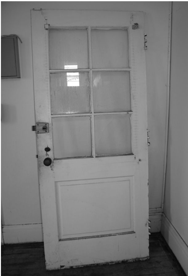
FIGURE 40. One of the original front doors.
