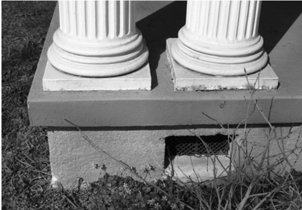
FIGURE 35. View of typical column plinths.
