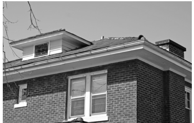
FIGURE 48. View of front dormer and capped chimney.
