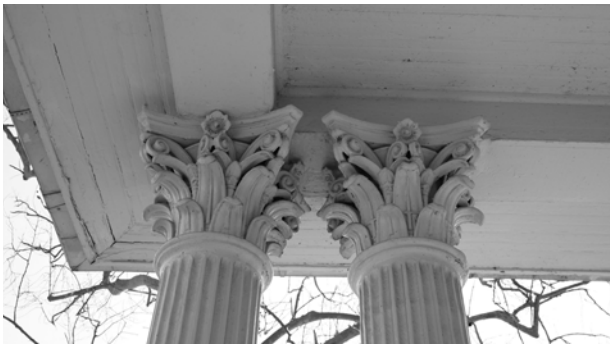
FIGURE 34. View of typical column capitals.
