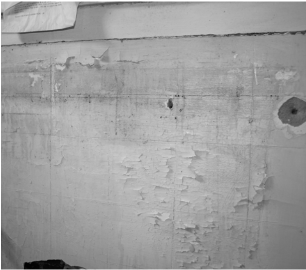
FIGURE 55. View of scored plaster wainscot in Room 103.
