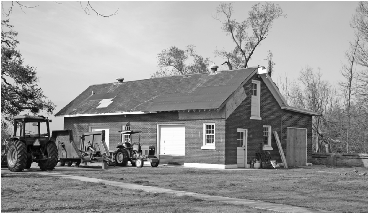
FIGURE 25. View west of maintenance building. (NPS, 2006)
