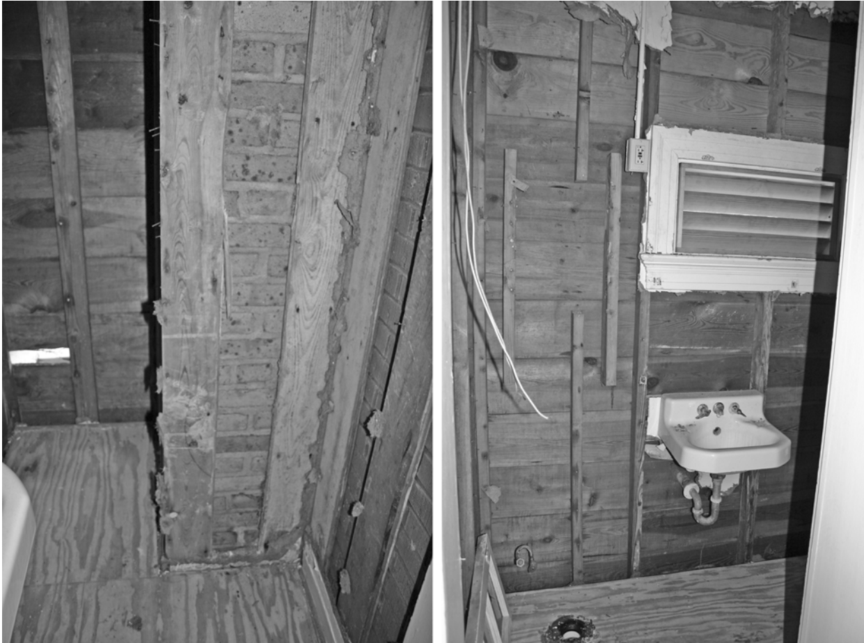
FIGURE 71. View northeast (left) and north (right) in Room 105. The odd framing visible in the right-hand image was probably to accommodate a wall-hung toilet tank.
