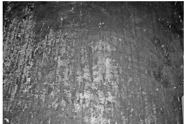
FIGURE 53. Oak flooring in Room 103 with mastic from vinyl floor coverings.
