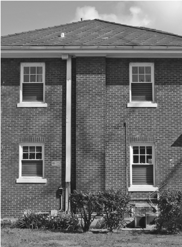
FIGURE 51. View of southwest chimney.
