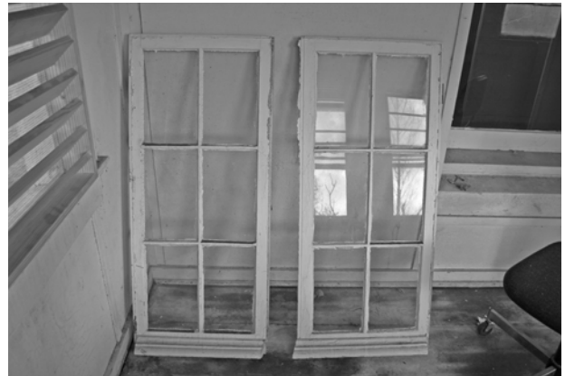
FIGURE 38. One of the surviving pairs of original sleeping porch windows.
