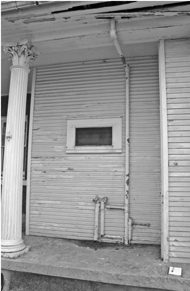
FIGURE 46. View of added bathroom.
