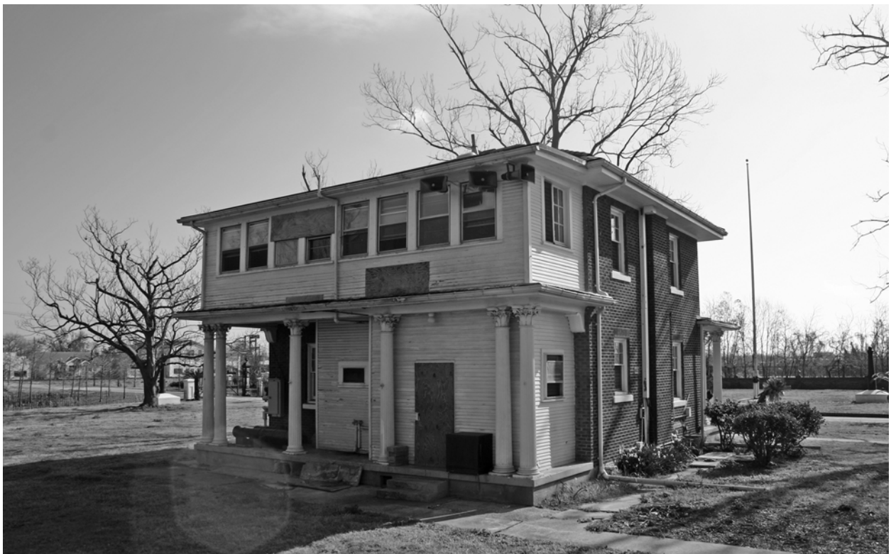
FIGURE 27. View east of Lodge. (NPS, 2006)
