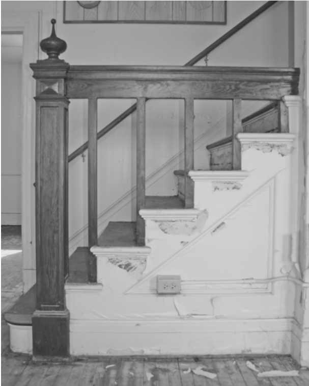
FIGURE 61. View of staircase in Room 101.
