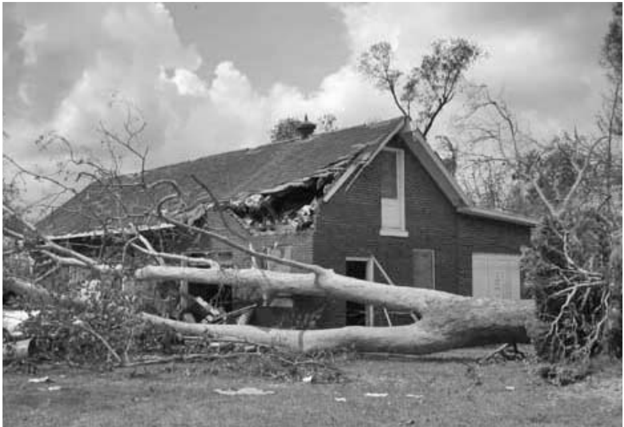
FIGURE 20. View of garage after Katrina. (JELA Coll.)
