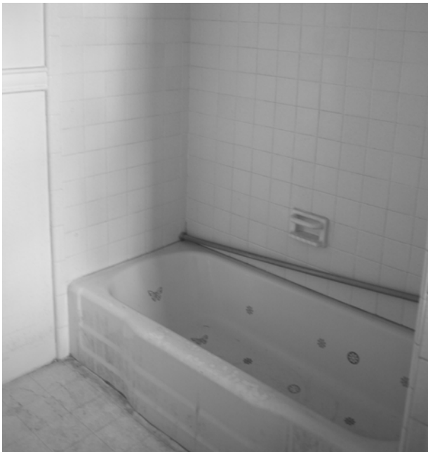
FIGURE 65. View of shower in Room 203.
