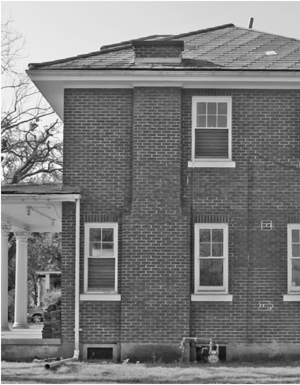
FIGURE 50. View of northeast chimney.
